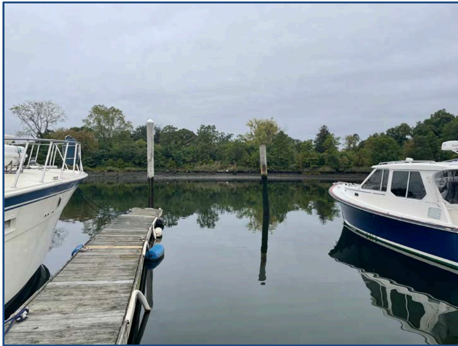
Photograph 1 – Pile number 44 is outlier in pile layout; only area with a tie off pile
