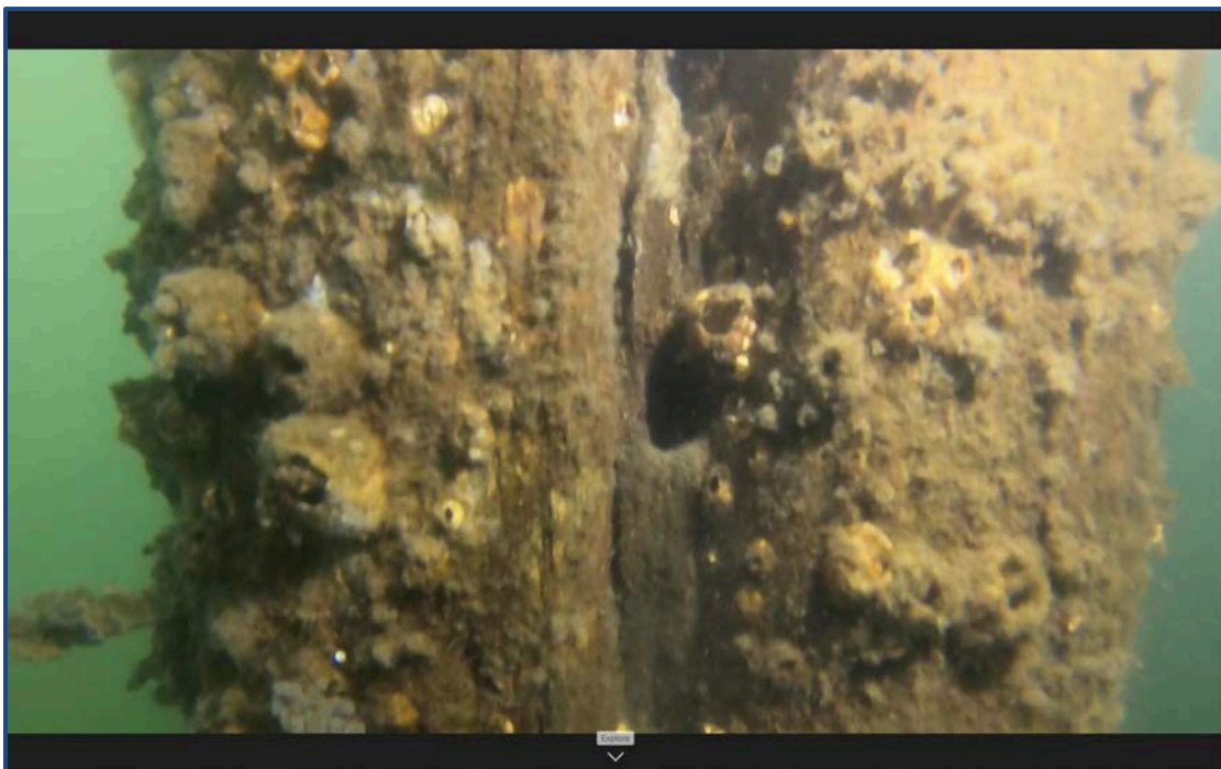
Photograph 6 – Marine borer damage in pile
