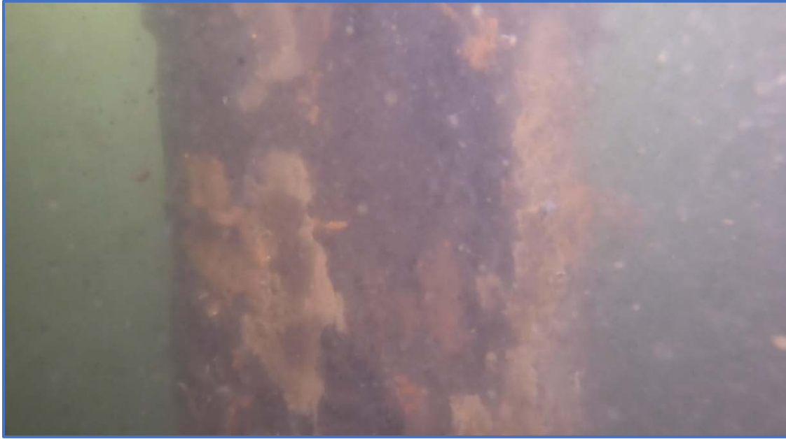
Photograph 3: Typical marine borer damage to pilings listed as Poor/Serious
