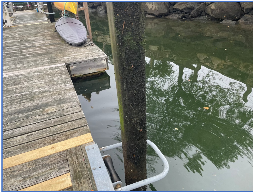
Photograph 5: Typical wear and tear from pile guide
