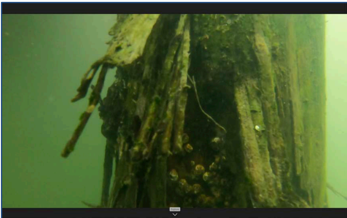
Photograph 8 – Severe ice damage in pile 5' below Mean High Water
