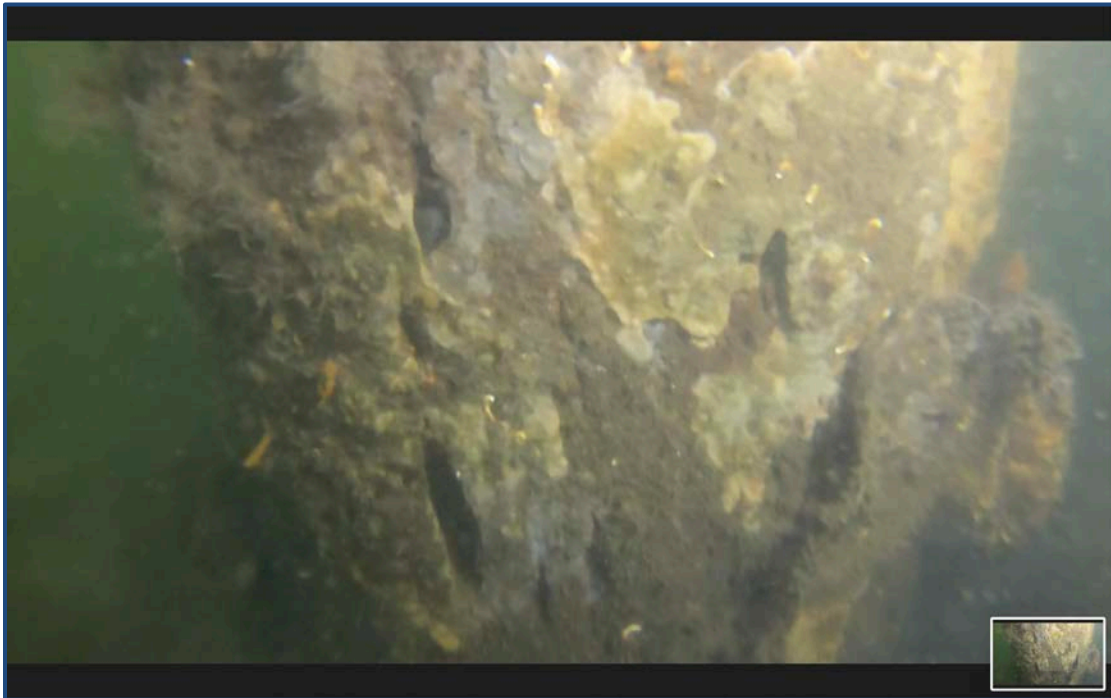
Photograph 7 – Significant marine borer damage in pile
