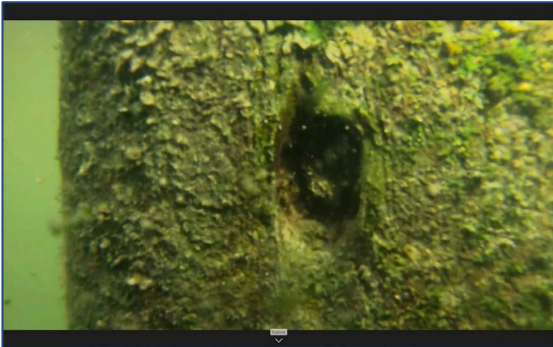
Photograph 5 – Marine borer damage at a knot in the pile
