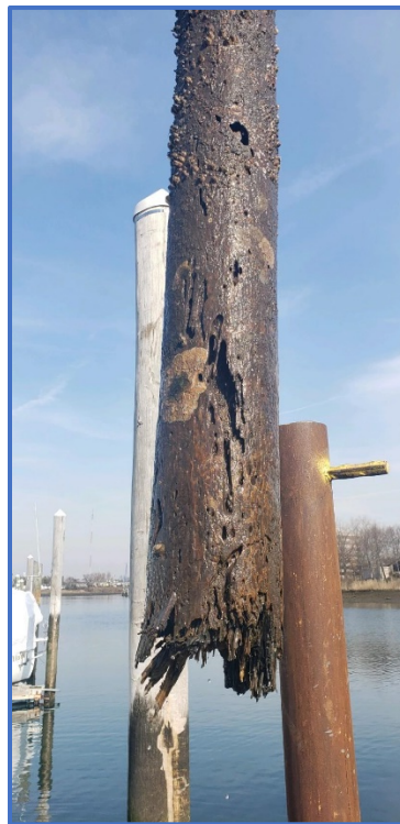
Photograph 4: Broken Pile provided by SCYA
