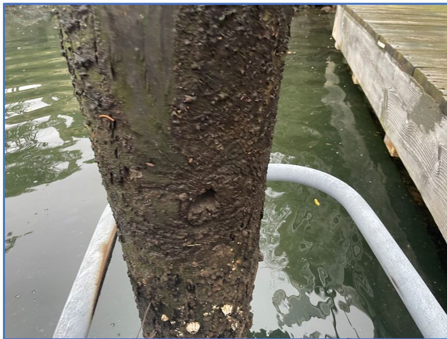
Photograph 2: Typical marine borer damage at knot of piling
