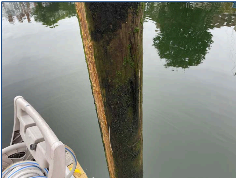
Photograph 2 – Typical abrasion damage from pile guide
