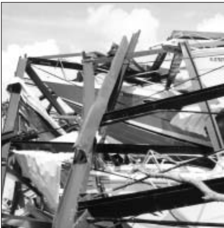
High-rise storage racks can be toppled by a storm's high winds. If possible, put your boat on a trailer and take it further inland.
